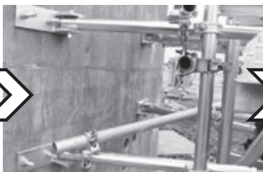
壁つなぎ取付け
